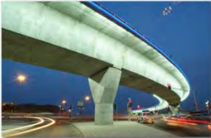
Gilot Bridge Illumination
