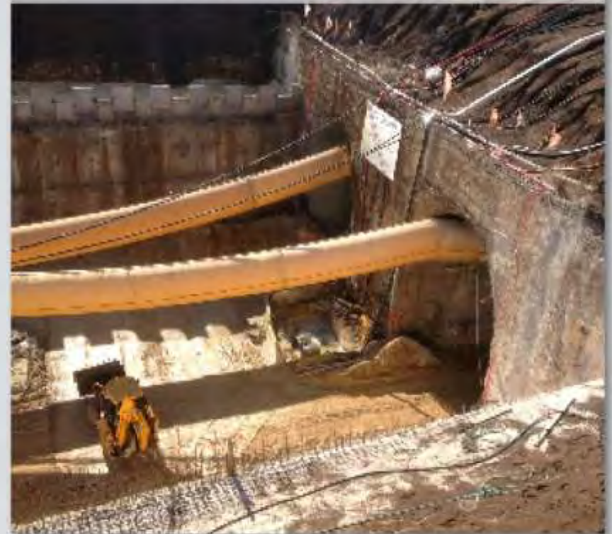
Gilon railway tunnel site
